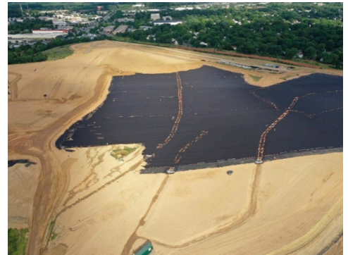
Phase VI after liner installation
