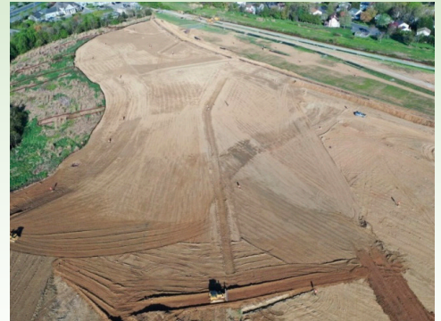
Phase V and VI after waste excavation and grading from April 2024
